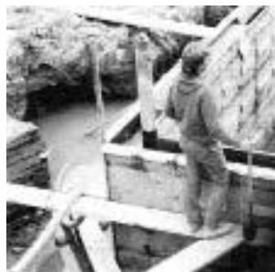
Figure 5. Too late in the excavation, Design Extension and Builders discovered a spring in the daylight basement area of a foundation. The solution was to backfill both sides of the frost wall with crushed stone for continual drainage, create several bond-outs through the footing to equalize inside and outside water pressure, and provide a permanent 6-inch drain pipe to direct the spring water away from the building.
