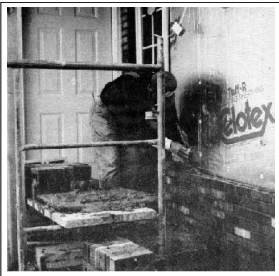
A brick veneer goes right over insulating board and wood studs. The veneer protects the house from wind.
