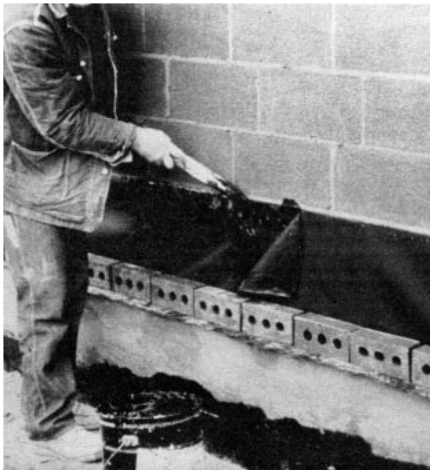
Figure 7. The bricklayer laps the flashing and seals the joint. Loose bricks hold the flashing in place and ensure that it won't get bunched up in the wall or torn during construction.
