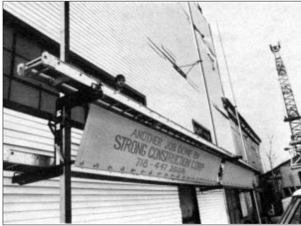
Figure 6. Pump jacks are easy to set up. This assembly from Alum-a-Pole features a protective screen that can display company advertising.
