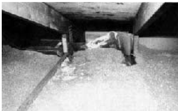
Figure 4. These insulation baffles (left) are ineffective since they are misplaced and damaged from heavy condensation. The baffles should be rigid and placed as shown (right) to keep wind from blowing under the insulation (windwashing), causing condensation, mold, and mildew at the ceiling corners.
