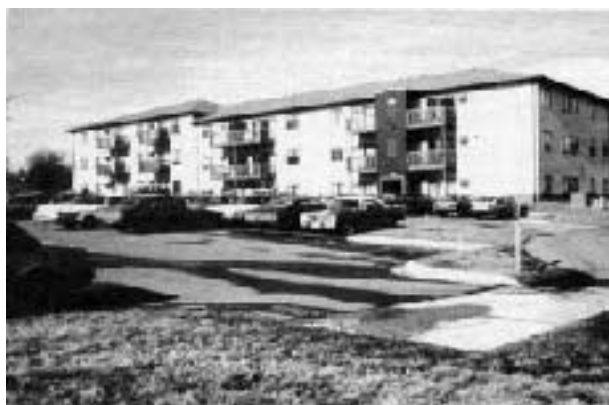
obvious that the building was tight enough that it needed continuous ventilation in each unit. Sure enough, a survey of the occupants revealed that over half rated their apartments air quality fair to poor.
