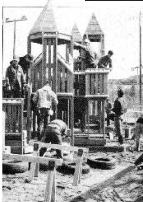
On projects like this one (left) in Buloxi, Miss., Segal finds it's safe to use only dense, full dimension, kiln-dried lumber that's been treated with CCA-C or CCA-B (avoiding the A, or generic, variety) and then redried after treatment.
