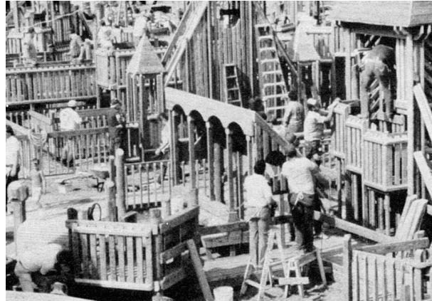
Segal's playgrounds always draw on local citizens as the labor pool. One project involved 1,750 workers. But most, like the one above, in Grant's Pass, Ore., have modest sized crews.
