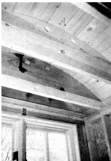
Figure 2. Two-by-fours were added to the bottom edge of each 2x12 curved rafter. Note the 2-inch vent holes drilled in each rafter to provide ventilation into the main attic.
