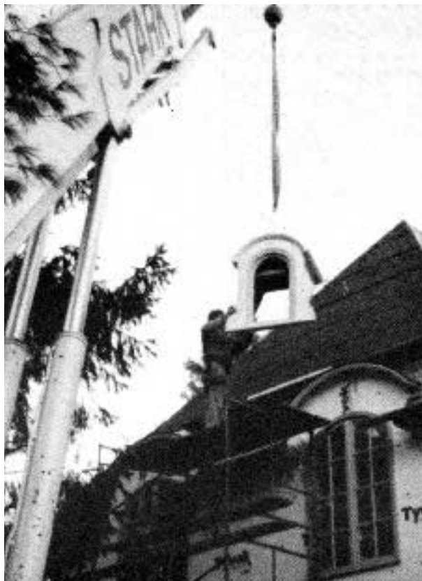
A shop-built curved-top dormer is set with a crane. The opening in the roof has been sheathed over to guard against weather, and it will be cut out after the dormer is in place.
