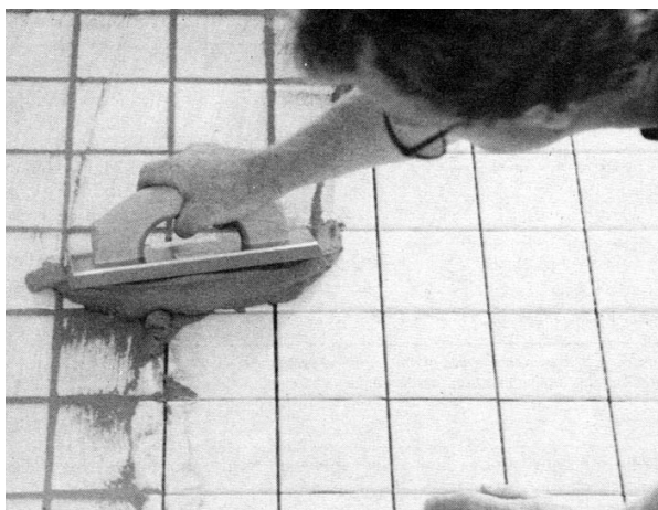
With plenty of fresh grout under the trowel, the author forces the material into the joints. The key is to apply ample force and work the trowel from several directions, holding it at 15 to 25 degrees.
