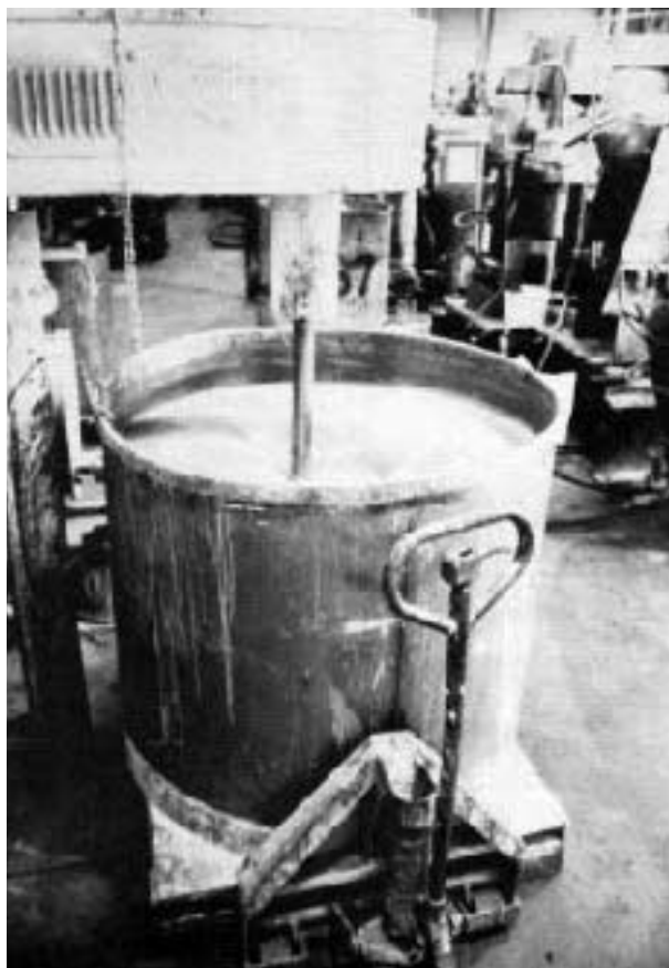
Paint manufacturers mix pigments and resins and thin with solvents in huge vats like the one above. However, in low-VOC oil paints, solvents are replaced in part with solids, yielding heavy and thick formulations.
