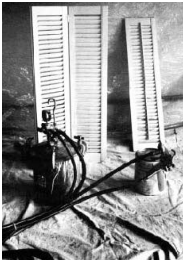
Shutters and similar woodwork would ordinarily get sprayed with several thin undercoats and an oil-based top coat. But low-VOC oil-based enamels are very difficult to spray, and water-based coatings lack the needed durability.
