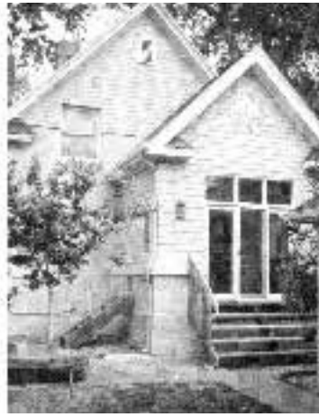
Figure 4. Matching existing materials is vital to making an addition blend in, but it can overwhelm the budget. In replacing the wood sleeping porch (left) with a breakfast room (right) on this brick Victorian, the solution was to use salvaged brick on only a small part of the addition—in the base and belt course—and shingles on the rest. The flare where brick and shingles meet imitates a detail found at the top of the first-floor brick walls on the front of the house. Since both the brick and gable end shingles of the original house were painted, extending this single color to the addition was an important factor in tying everything together. The diamond-shaped window atop the addition brings high sunlight into the vaulted breakfast room, and adds a distinctive touch.
