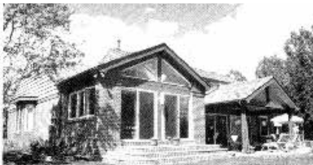
Figure 3. Matching the existing roof style often means using "cross-gables" at the same pitch, rather than taking the easy route with a shed roof. In replacing this shed patio cover (left), we brought the family room addition starts out with a shed roof, but then makes the transition to a gable to form the patio cover. The 12-foot ridge height lets south sun penetrate into the family room in winter, while shading the high summer sun. The kitchen wing has trapezoidal windows with no overhang to allow maximum penetration of sunlight into the 21-foot deep space.
