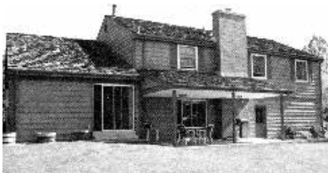
Figure 3. Matching the existing roof style often means using "cross-gables" at the same pitch, rather than taking the easy route with a shed roof. In replacing this shed patio cover (left), we brought the family room addition starts out with a shed roof, but then makes the transition to a gable to form the patio cover. The 12-foot ridge height lets south sun penetrate into the family room in winter, while shading the high summer sun. The kitchen wing has trapezoidal windows with no overhang to allow maximum penetration of sunlight into the 21-foot deep space.
