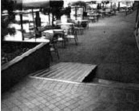
If The Americans with Disabilities Act passes, it will mandate changes in the design and construction of commercial buildings and apartments. Installation of access ramps may be required by Federal law.
