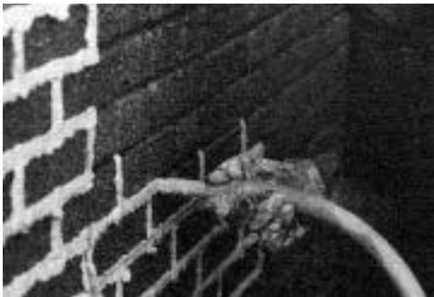
The mason injects repointing mortar in joints that have been prepared with a grinder.
