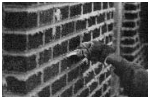
After the applied mortar is partially dry, a second mason comes along and strikes the joint.
