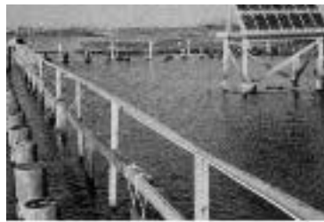
A bank of photovoltaics sends a small electrical charge to wire mesh forms hung in the seawater from wood frames. Minerals contained in the seawater are deposited on the wire mesh, thereby "growing" a wall.
