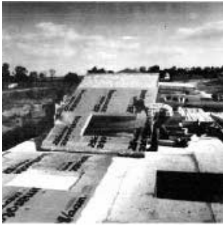
Figure 2. The framing crew places panels as close as possible to their location (top), then raises and nails them in place (bottom).
