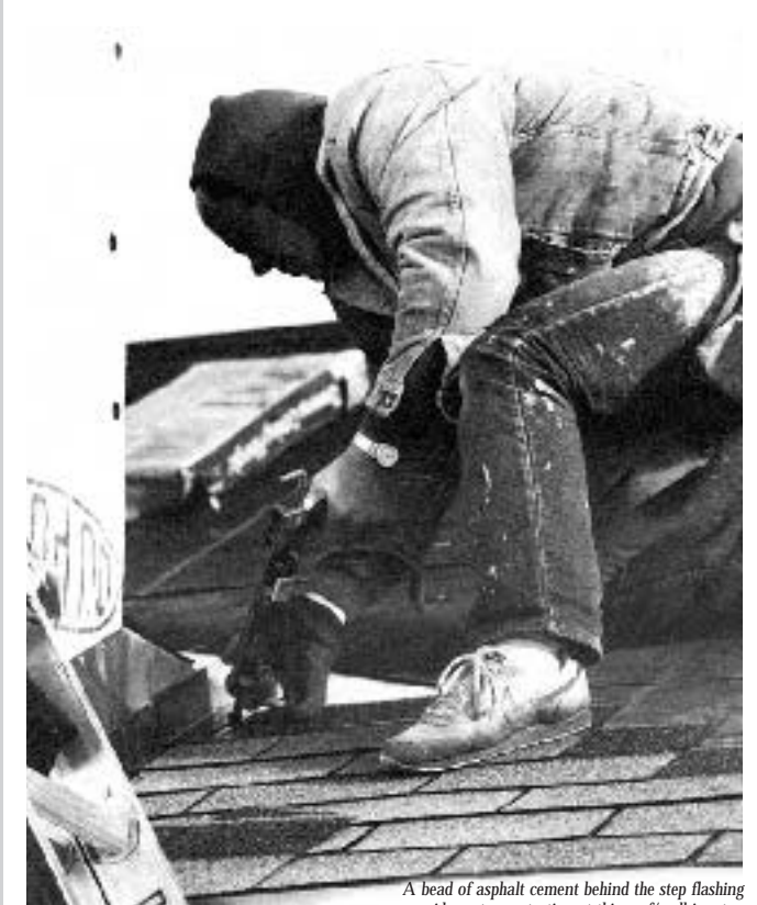
A bead of asphalt cement behind the step flashing provides extra protection at this roof/wall juncture.
