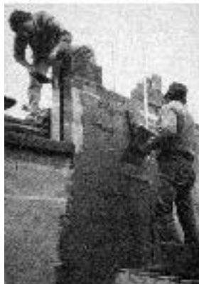
Sparfil's new parging system: After nailing the fiberglass mesh to the block, a worker uses a heavy-nap roller (top) to thoroughly wet the wall. Next, a carpenter works the parging through the mesh (bottom) with a steel trowel. Later, he'll apply a second parging coat and smooth the finish with a rubber squeegee trowel.
