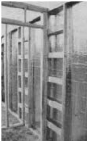
Figure 4. The insulation and vapor barrier are not penetrated by electrical boxes or plumbing. Interior partitions are tied to nailers.
