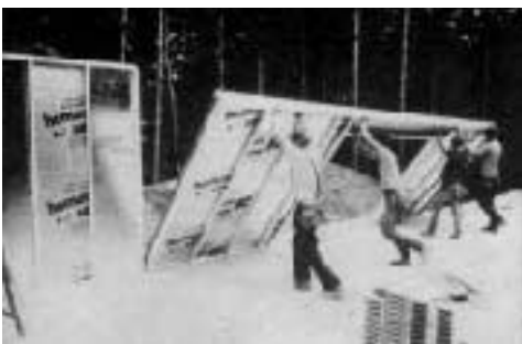
Figure 2. The walls are light and easy to lift into place. A conventional 2x8 upper top plate splices the sections together.
