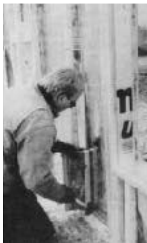
Figure 3. Foam strips are tapped into place against each stud to hold the large panels of foam tightly against the outer 2x2 flanges. This makes a tight seal and leaves room on the interior for plumbing and wiring.
