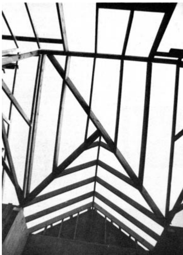
The extended valley rafter (top) provides a sturdy structure since it bears on the ridge and the wall top plate. The side view (bottom) shows the treatment at the eaves and gable end.
