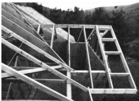
The extended valley rafter (top) provides a sturdy structure since it bears on the ridge and the wall top plate. The side view (bottom) shows the treatment at the eaves and gable end.
