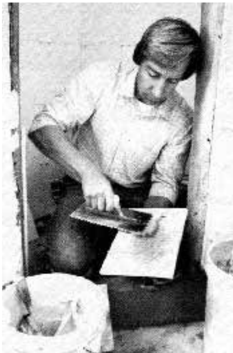
Figure 5. Here, the author butters a 12-inch Thassos marble tile with a 1/4-inch notched trowel. This Greek stone is stark white, requiring the use of white thinset. It will be set in place in the shower just 1/16 inch from neighboring tiles using small, wedged-shaped plastic spacers.
