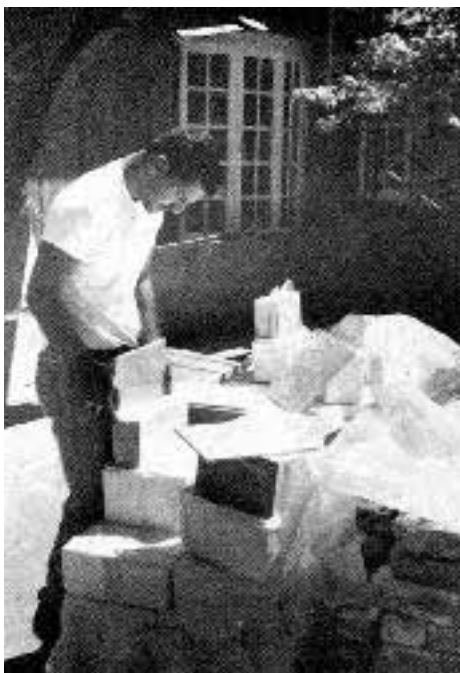
Figure 2. With marble and granite, it's important to inspect carefully and sort the material because of the wide variations with any batch. The tile setter's judgment determines which individual tiles will look good together in terms of their shading, veining, and grain direction.
