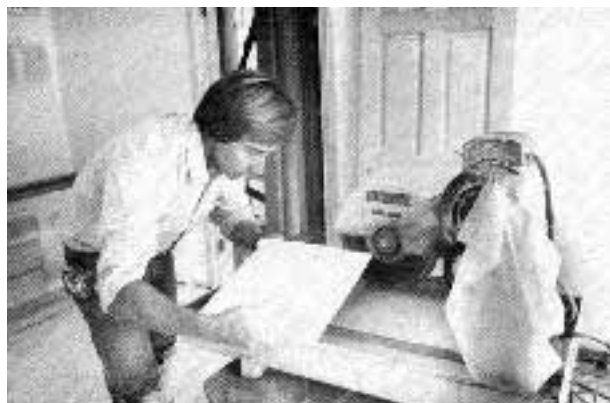
Figure 4. The author freehands a bevel cut on a marble tile using a water-cooled tile saw with a diamond blade. Granite is handled the same way, although cutting (and shaping and polishing) go slower because of the density of this volcanic stone.
