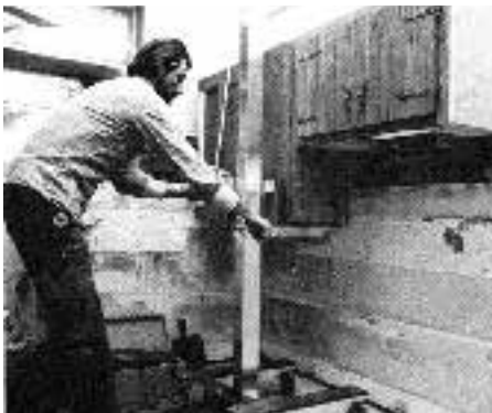
Figure 4. Gil-Lift is a four-wheeled dolly that can jack a wall cabinet up, level it, and hold it in place for attachment. Hoists like these are ideal for one-man cabinet installations.
