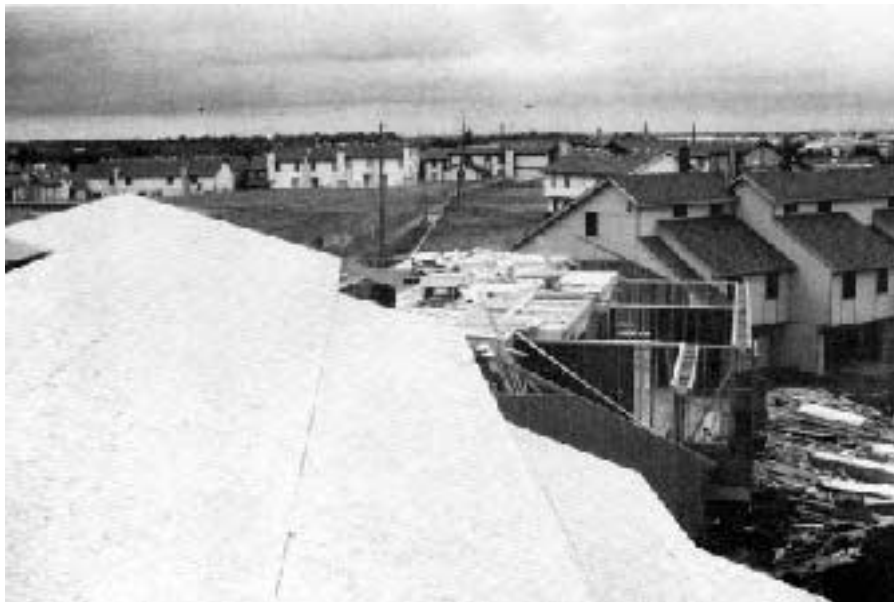
In some areas, OSB is replacing plywood as the leading choice for roof sheathing and subflooring.
