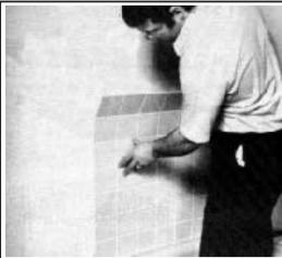
Pregrouted tile. American Olean's Redi-Set 100, shown above, has made a name for itself because it is a time-saver. The glazed, ceramic tile is manufactured in sheets that cover 2 square feet (4-1/4-inch tile) or 2.14 square feet (6x4-1/4 inch tile). The sheets are pregrouted with white silicone rubber grout. As soon as the tile is installed, the joints between sheets can be grouted to match. This eliminates the need for the tile setter to return to the site.
