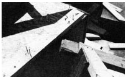
Figure 1. Wind uplift pulled these studs away from the bottom plate. End-nailing alone offers little resistance to tensile forces.
