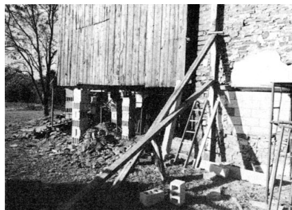
Figure 4. Shoring existing walls ensures that they are not damaged by stresses caused by work on nearby areas.
