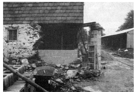
After jacking and blocking the timber frame (top right), new footings are poured. A block foundation is put in place (bottom right) and the original stones are used again to face the wall. The frame is eventually lowered back down.
