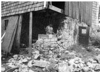
Figure 5. When working in a corner, drop a plumb line from the corner of the frame to a masonry nail set into the footing. Then, run strings horizontally to the existing stonework and blend in the new section of wall.
