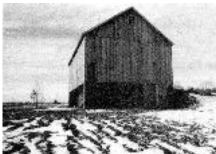
Figure 1. A Pennsylvania bank barn gets its name from the earthen embankment on one side. This design allows ground-level access to both the first and second floors. Stone foundations and stone walls are common.
