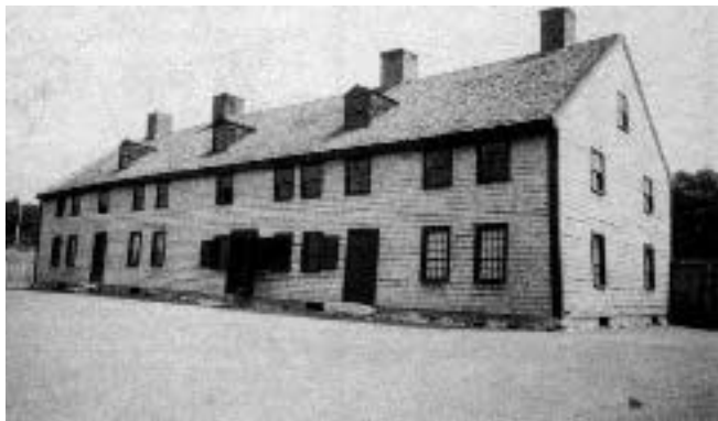
Figure 1. These four brick chimneys at the Fort Western Barracks museum had persistent leaks.
