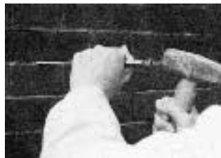
Figure 3. A hammer and plugging chisel may be needed when the mortar is too hard to rake out.
