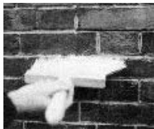
Figure 6. Use a brush to give joints a "weathered" look.
