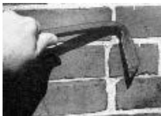
Figure 2. The thin blade of a mortar rake slips into narrow joints without damaging them.
