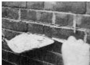
Figure 4. The narrow pointing trowel slices a ribbon of mortar off the large pointed trowel and places the mortar in the joint.
