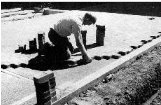
Figure 5. With concrete pavers, a 6- to 10-inch granular base will handle most driveway loads, but if you expect large trucks on the driveway, put in a 12- to 14-inch base. The shape and thickness of the paver affects its load-carrying characteristics.
