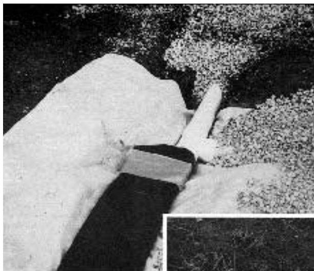
Figure 4. Fin drains can be placed horizontally or vertically in the trench on the side of the driveway to collect water and conduct it to a drain (inset). The filter fabric prevents clogging.
