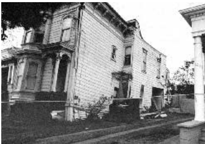
The unbraced cripple walls of this West Oakland home succumbed to the 7.1 quake of Oct. 17, leading to their collapse at the rear of the house. Shearwall bracing and substructure diagonal braces would have given this home a better chance.
