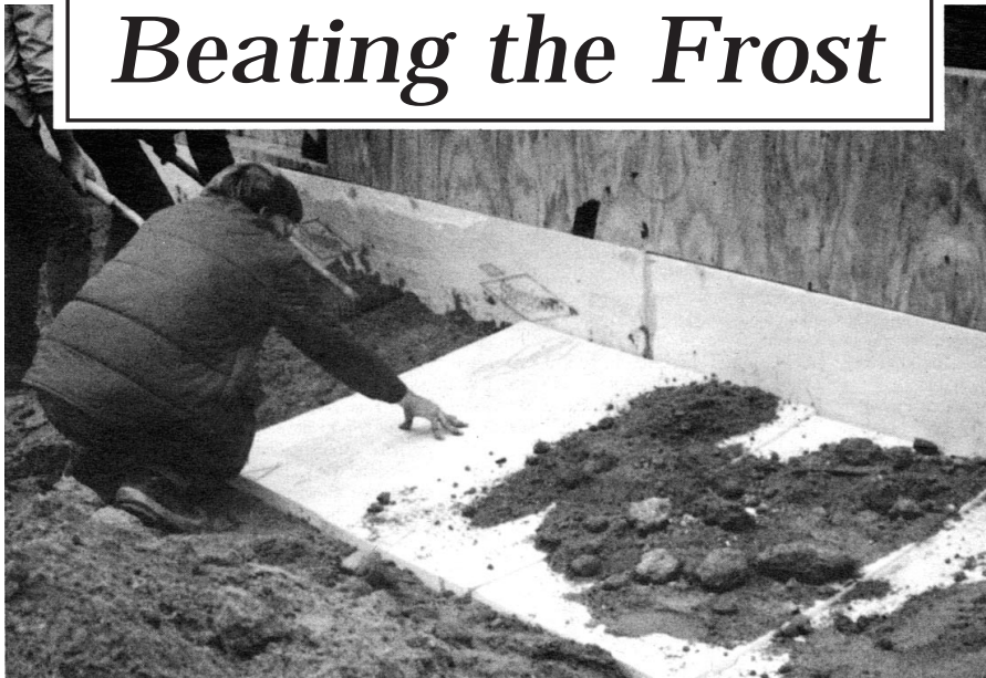
A shallow layer of topsoil is shoveled onto the 2-inch polystyrene "skirt." The rigid insulation is sloped slightly away from the house to keep the soil dry around the foundation and slab – a key to preventing frost heaving.
