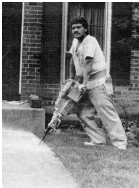
Figure 2. A gas-powered rotary drill takes 20 seconds to go through a 5-inch slab. A star or ball bit on the drill leaves a clean hole, ready for patching.
