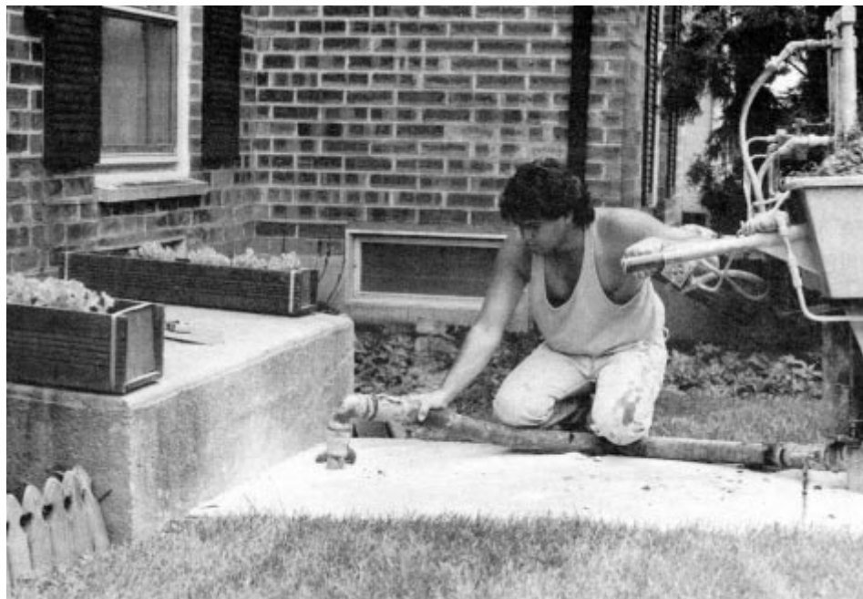
A worker injects grout beneath a concrete walkway that has cracked and settled. This will restore it to its original grade.
