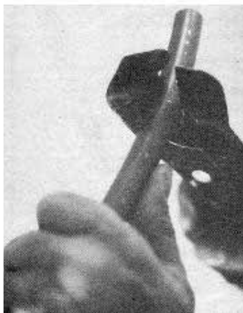
Figure 4. Hand-held cutters cut PB piping to length.
