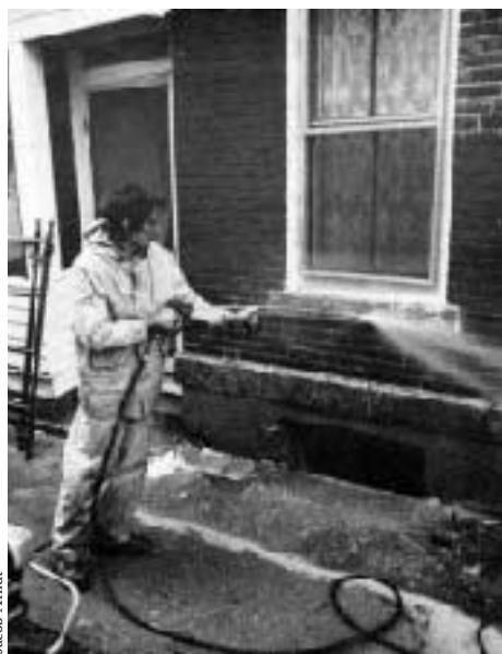
Figure 1. A rented pressure wand can be used to remove peeling or loose paint.
