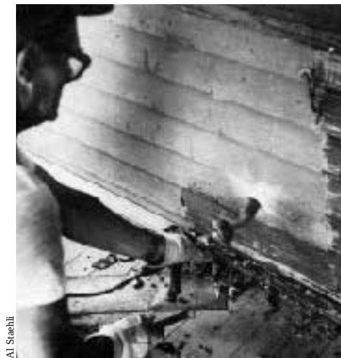
Figure 3. Ed Bell & Sons crews work quickly using light, hand-held torches fed from an LP tank. A rigorous safety program safeguards against fire.
