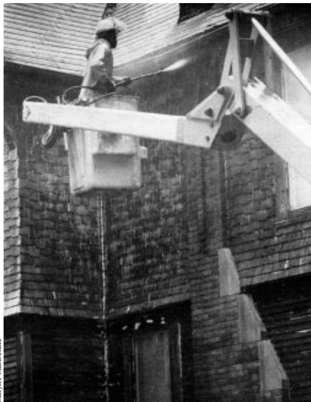
Figure 2. The worker in the bucket truck sprays a water rinse on a building that has been cleaned with caustic stripper. Unfortunately, the caustic runoff discolored the brick chimney. To avoid this, test the effects of chemical cleaners on all nearby materials.
