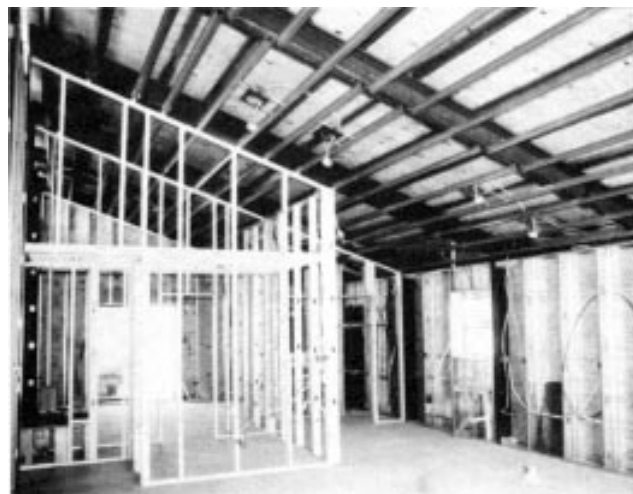
Figure 2. Interior walls are made from 3-5/8-inch metal studs, the exact dimension of a 2x4. Roof purlins that run perpendicular to the steel are 2-1/2-inch-deep hat channels, spaced 2-feet on-center.
