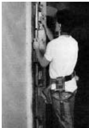
Figure 2. One-piece mortising templates such as this Porter-Cable 59380 can be used on an installed jamb.
