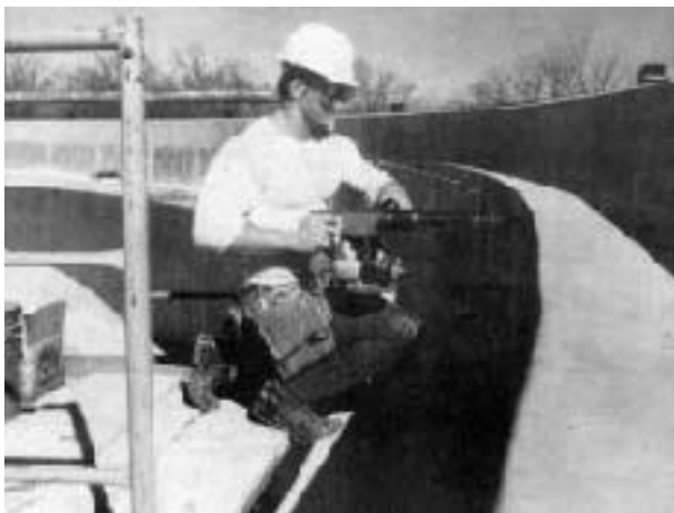
Figure 2. The Hilti GP 22 gasoline-powered hammer drill is powered by a tiny Kawasaki two-stroke engine. This makes it ideal for remote sites.
