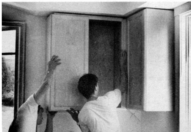
Figure 5. After checking measurements, the author rips a filler strip for the corner cabinet (above left), then glues and screws it to the cabinet (above). With the cabinet held temporarily in place the author checks the fit against the blind cabinet (left).
