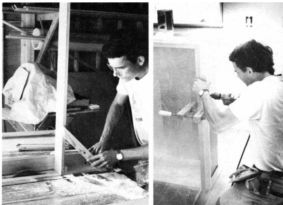
Figure 5. After checking measurements, the author rips a filler strip for the corner cabinet (above left), then glues and screws it to the cabinet (above). With the cabinet held temporarily in place the author checks the fit against the blind cabinet (left).
