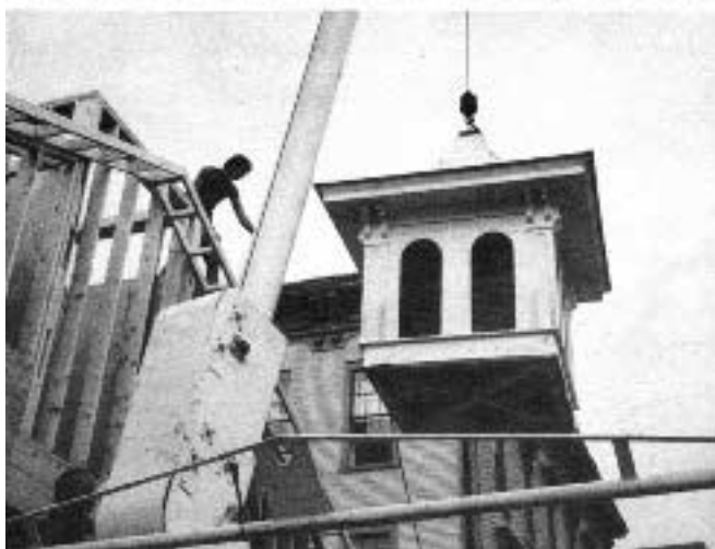
For roof framing, the author cut curved rafters from two layers of \frac{3}{4} -inch CDX plywood. The louvered openings in the base of the cupola are made from stock rectangular shutters overlaid with curved trim (top). Above, a crane picks up the cupola by its peak to set it in place.
