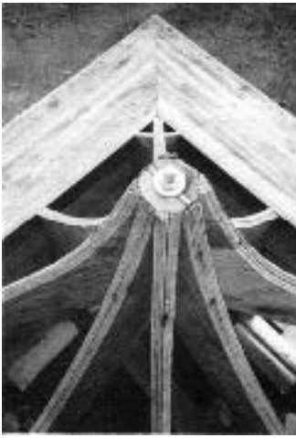
The rafters butt an octagonal ridge block glued up from two 24-inch-long 2x4s with 1/2-inch plywood strips sandwiched in between. A threaded rod, used for lifting the cupola, runs up through the center of the block.
