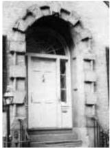
The doorway to this brownstone in the Beacon Hill section of Boston suffers from just about every brownstone failure. Many of the bricks are discolored from salt and are spalling from moisture. In other sections, large chips of stone have fallen away.
