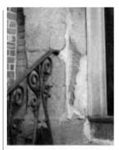
Water has caused the ironwork to rust and expand where it enters the brownstone trim, which has caused the stone to burst.
