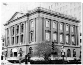
This stately Boston brownstone built in 1869 required extensive repairs. Restorers cut back its severely deteriorated trim and many of the blocks to solid stone and rebuilt the areas with tinted cement. The building, originally the Museum of Natural History, now houses a clothing store.
