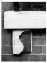
Painting over brownstone will not stop its deterioration. The crumbling stone should be removed and replaced with an appropriate cement patch.
