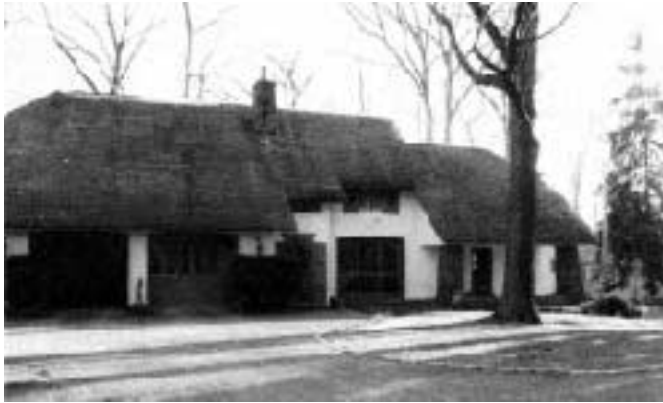
This carriage house is part of an estate built in Convent Station, N.J., for George M. Allen, who was obsessed with English history. The buildings were designed by architect Charles I. Berg to resemble the thatched roofs common on the English countryside.
