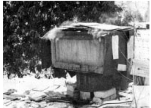
Shingles were placed upright on a rack in the box, while a small propane heater boiled a small amount of water in the base.
