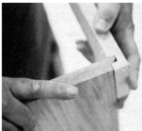
Figure 2. A tongue on the tread fits into a dado in the face of the riser, making for a clean, tight joint.
