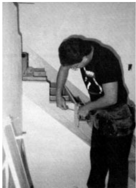
Figure 3. To make the joint between riser and open skirt as tight as possible, the author scribes the riser cut directly off the skirtboard; the line is then transferred to the front of the riser for cutting.
