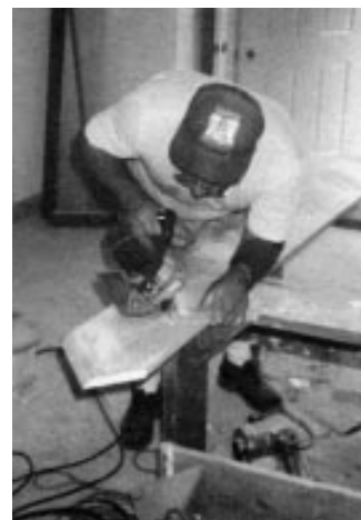
Figure 1. Here the author carefully cuts the open skirt using a Porter-Cable Saw-Boss, which tilts left like a worm-drive saw.
