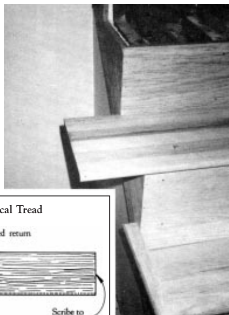
Figure 4. The upper tread is set snugly into place to mark the cut for the bullnose return. The lower tread shows the finished bullnose return (detail inset).
