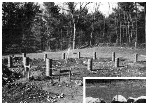
Figure 2. After placing the builders tubes and backfilling around them (above), the author used a transit to accurately mark the tubes for cutting at grade. Anchor bolts were placed (right) after the ready-mix truck filled the tubes.
