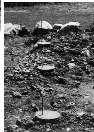
Figure 2. After placing the builders tubes and backfilling around them (above), the author used a transit to accurately mark the tubes for cutting at grade. Anchor bolts were placed (right) after the ready-mix truck filled the tubes.
