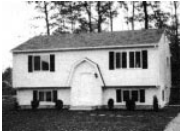
This partially finished house is one of two models sold by a Rhode Island builder for $95,000.
