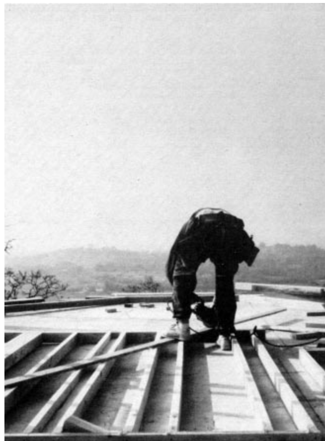
Figure 2. To speed up the process of cutting in sway (let-in) braces, framers hold the 1x in place with one foot and run the saw along each side. This short cut takes practice and caution.
