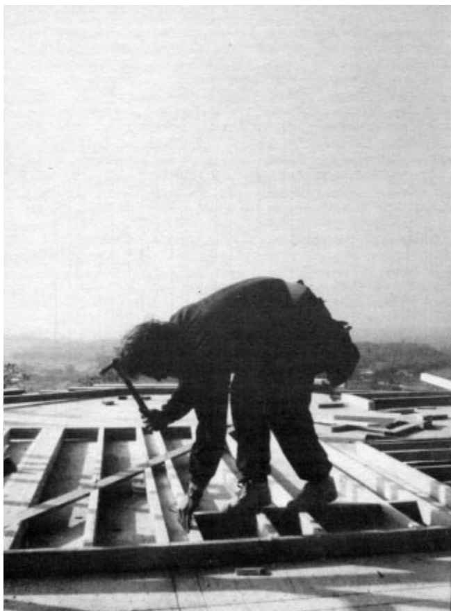
Figure 3. Blocking can typically be cut in place without measuring by laying the stock on the wall and eyeballing the saw blade.
