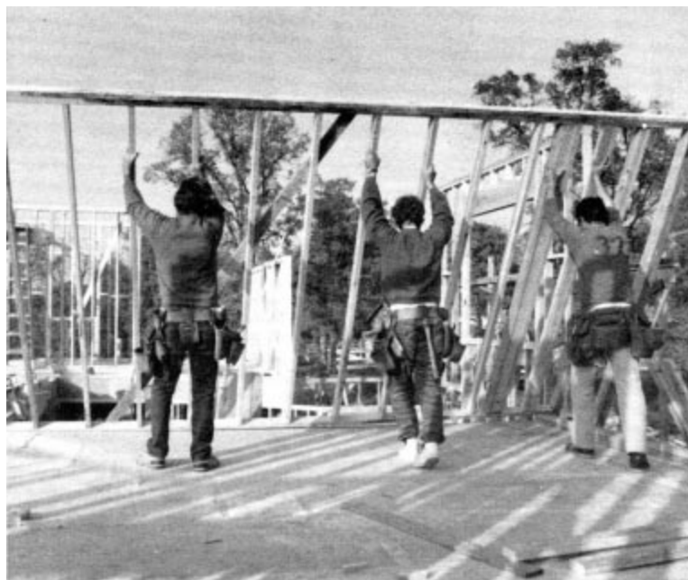
Following careful layout, walls are banged together and raised with assembly-line speed and efficiency.
