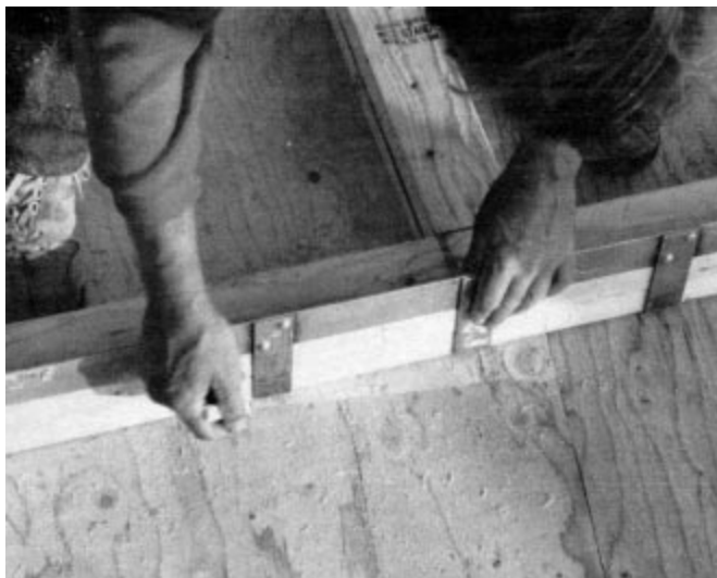
Figure 1. A layout stick eliminates the occasional errors that come from stretching a tape and having to pick out stud centers. It also saves the extra steps of squaring off marks and making Xs.
