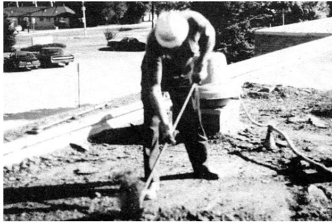
Figure 1. For clearing aggregate from a large area, most roofers use a spud bar.
