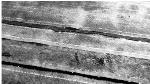
Figure 5. Fishmouths are found at seams and are usually due to installation problems.
