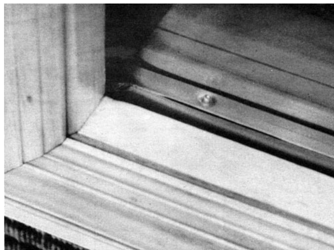
Figure 1. One way to tell that a window is gas-filled is by the plugged filling hole which is usually visible as a small nipple on the inside of the metallic edge spacer.
