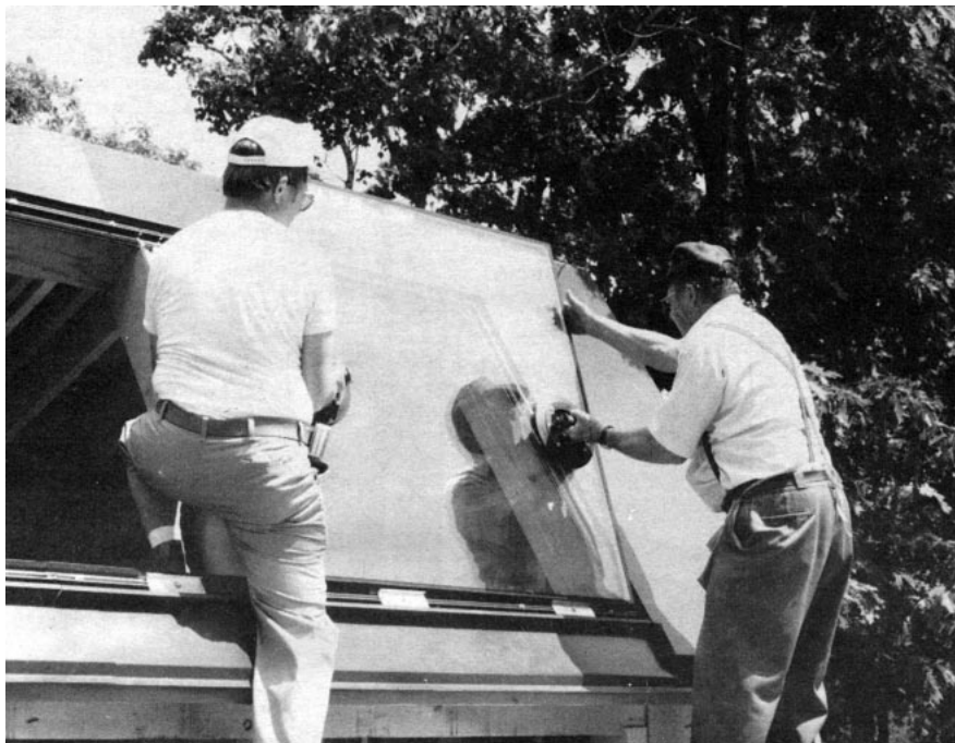
Workers set an insulated glass unit onto an extruded aluminum batten system. Suction handles help them maneuver the glass.
