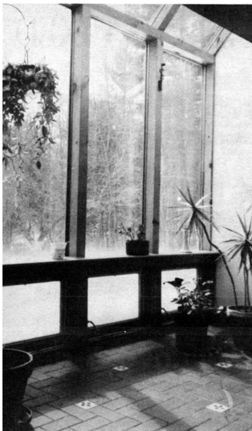
Figure 1. Glazing posts and rafters must be strong and dimensionally stable to prevent excessive movement. Douglas fir in Clear or B-grade is the author's favorite for sunspaces. The horizontal divider makes an attractive shelf.
