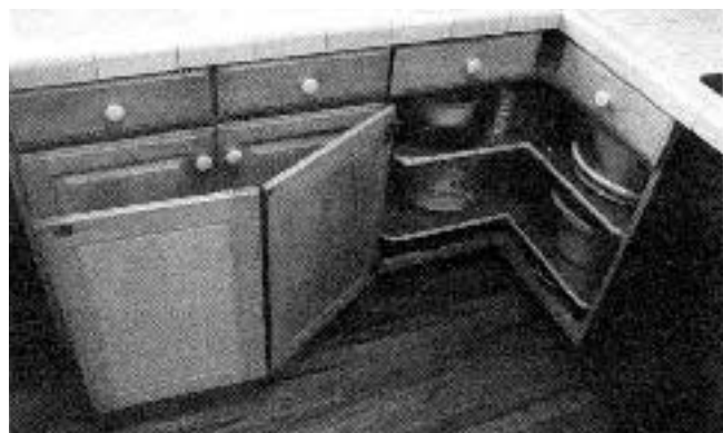
Figure 1. Free-hung, bi-fold doors often work well with a lazy Susan in an L-shaped cabinet. The more typical doors which attach to the shelves, look out of place in kitchens with overlay doors on the rest of the cabinets.
