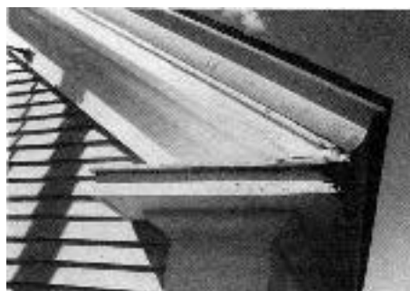
Figure 1. Squirrels chewed a hole into the joint where the rake molding meets the gable end return and the front crown molding.
