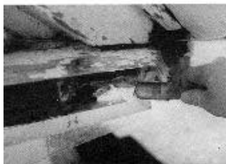
Figure 2. Wearing gloves, the carpenter works epoxy paste filler into the patch area with a putty knife.
