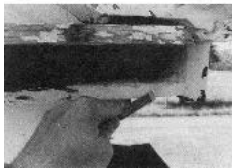
Figure 3. After the epoxy paste hardens, surfaces and edges are chiseled or rasped to match the adjacent wood.
