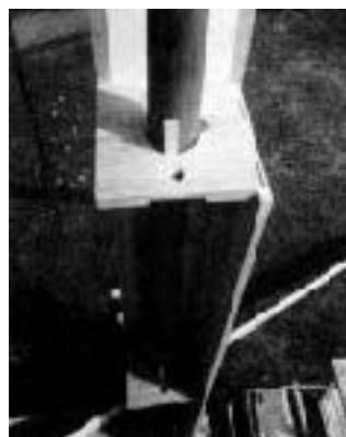
Figure 2. To provide a snug nailer for the wood column, the author slipped two plywood supports, one from each side, around the steel post. He nailed the supports together, then drove in wedges to secure them. Note the biscuit slots in the end of the pine 1x12 at right.
