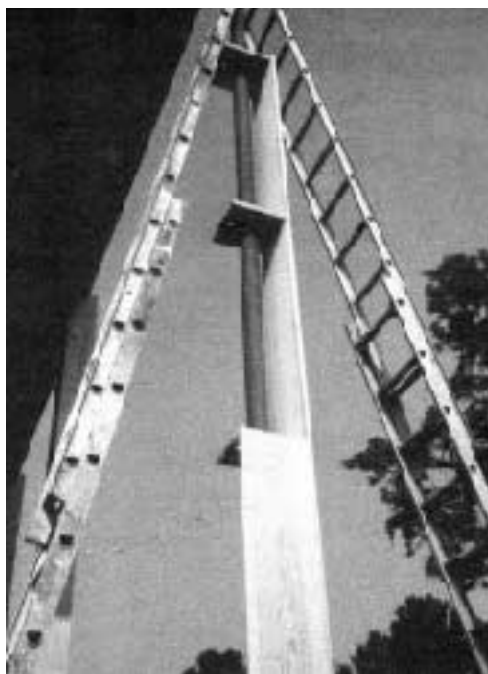
Figure 4. Lots of trips up and down the ladders made for slightly risky work.
