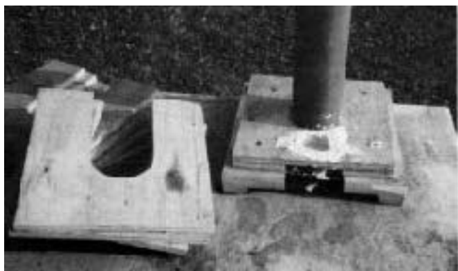
Figure 1. The columns rest on aluminum plinths (at right), slotted so they could be slipped around the steel posts. At left is a stack of the plywood supports the author devised for fastening the wood columns to the steel posts.
