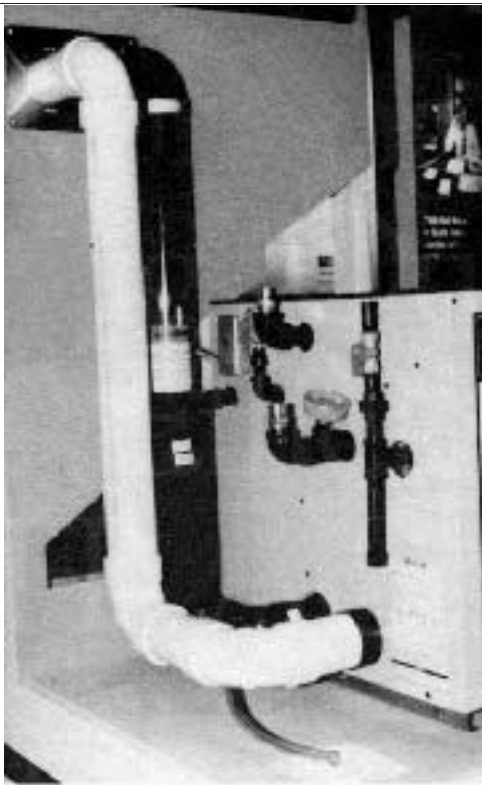
Figure 5. Corrosion-free venting. To prevent corrosion in a high-efficiency boiler, such as the Weil McLain GV model shown here, the venting system must be Ultravent or Plexvent high-temperature plastic vent pipe (the black pipe in the photo). Made of GE Ultem plastic, these vent systems can withstand temperatures up to 480°F. The white pipe is the fresh air intake, which is made of ordinary Schedule 40 PVC.
