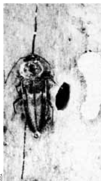
Old house borer larvae, at right, attack the sapwood of structural members. They may feed for three to seven years before emerging from \frac{1}{4} to \frac{3}{8} -inch exit holes as adult beetles, left.
